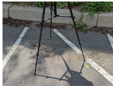
(e) H2 measuring asphalt surface material
